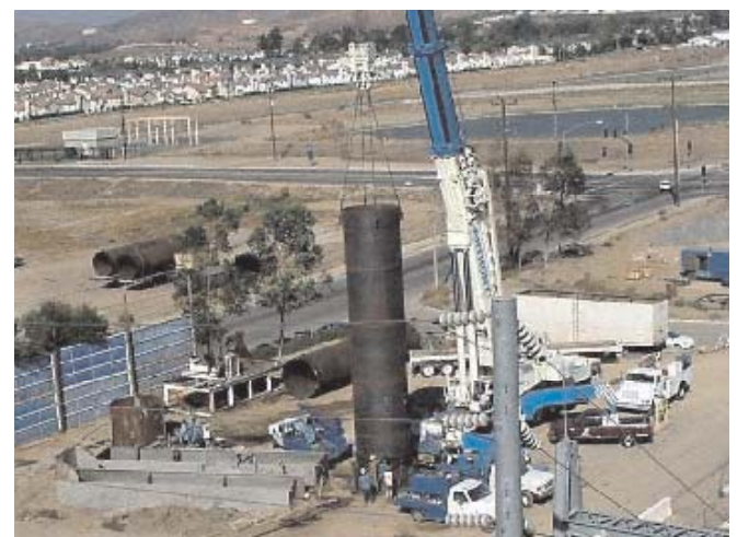
VERTREAT™ aeration shaft placement
