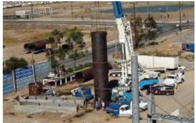
VERTREAT™ aeration shaft placement
