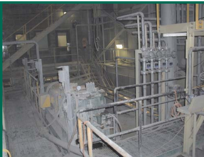
Paprilox® Retrofit of Existing Causticizers
